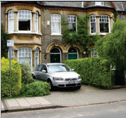
Front boundary removed for car parking
