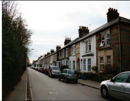
Brick detail painted over.
